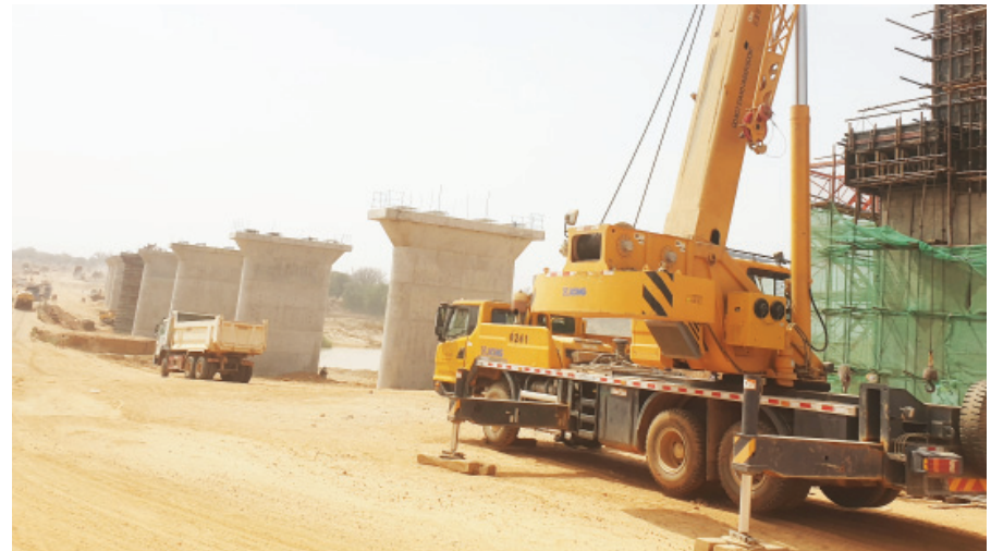
Some part of the completed project awaiting the rail tracks
