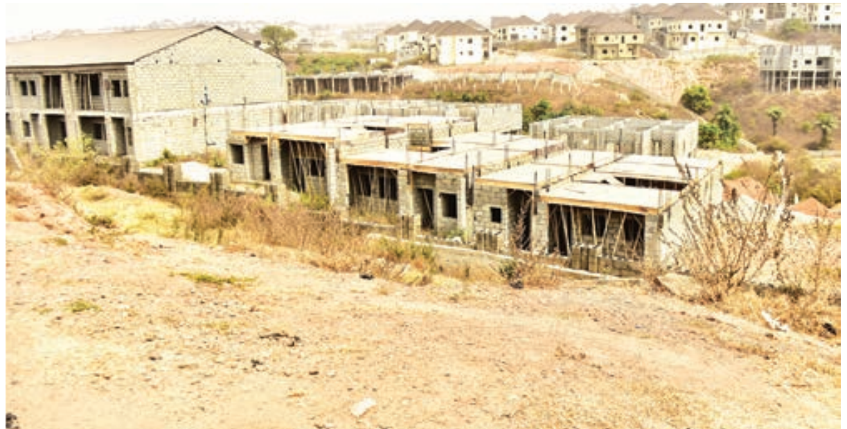
■ An estate under construction behind Mogadishu Cantonment, Asokoro, Abuja
