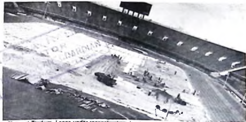
• National Stadium, Lagos under reconstruction. Inadequate facilities hinder performance
