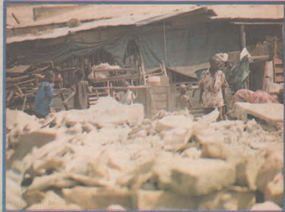
Children search through the rubble of their demolished homes in Nyanya..Friday
