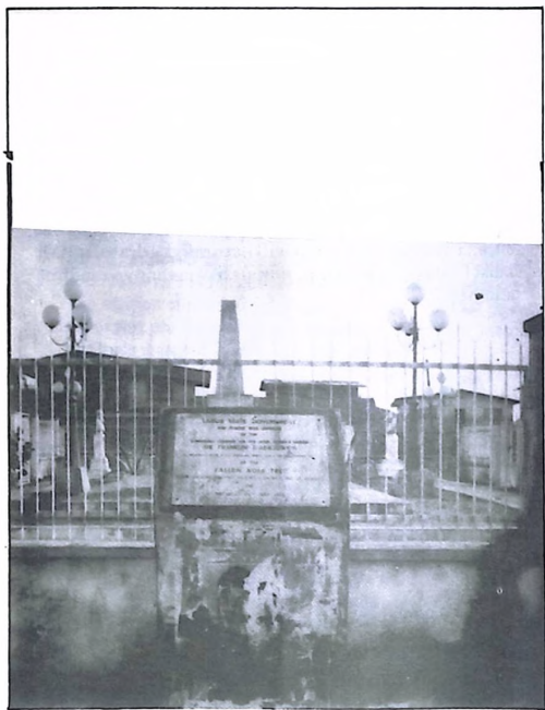
Erection on the site of the fallen AGIA TREE.
