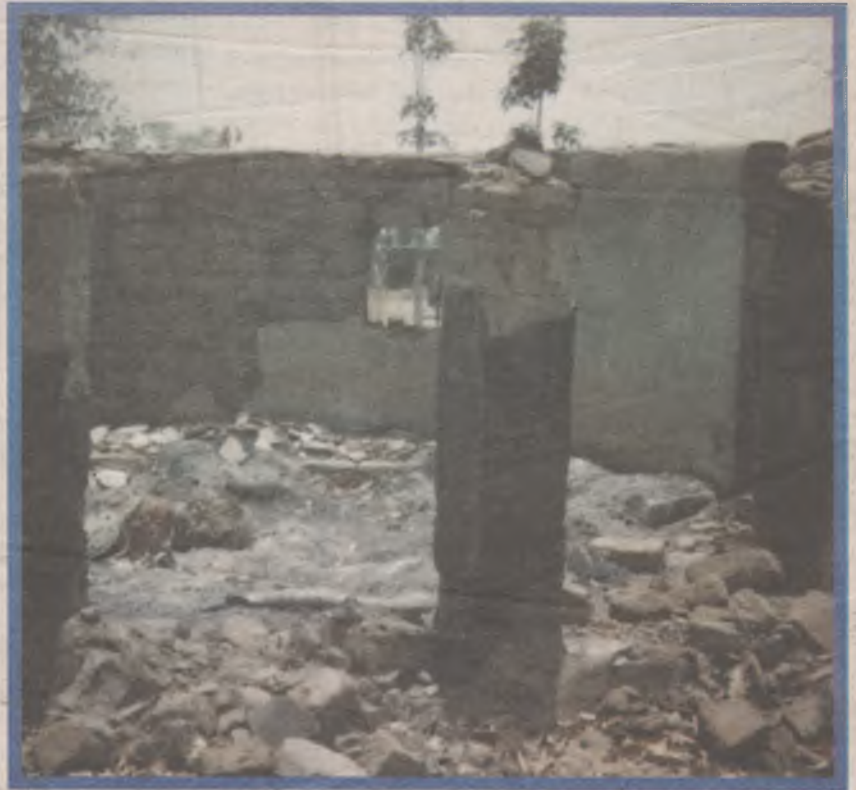
Destroyed buildings during communal clashes in Kwalla, Plateau State... last week
