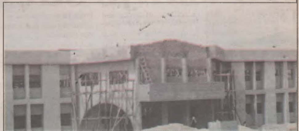
Gombe Radio and Television building under construction.
