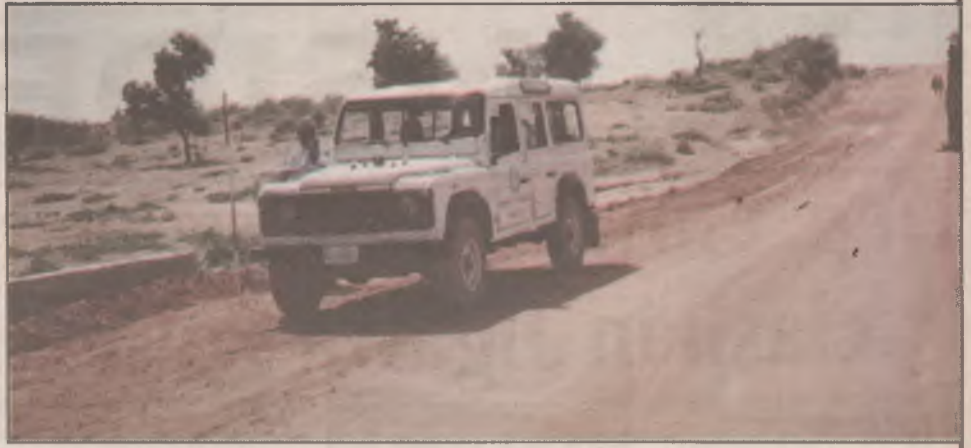
Gombe-Abba Junction-Hashidu Road, under construction by Abubakar Hashidu administration.
