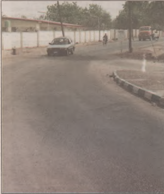
One of the township roads rehabilitated by Gov. Abubakar Hashidu administration.
