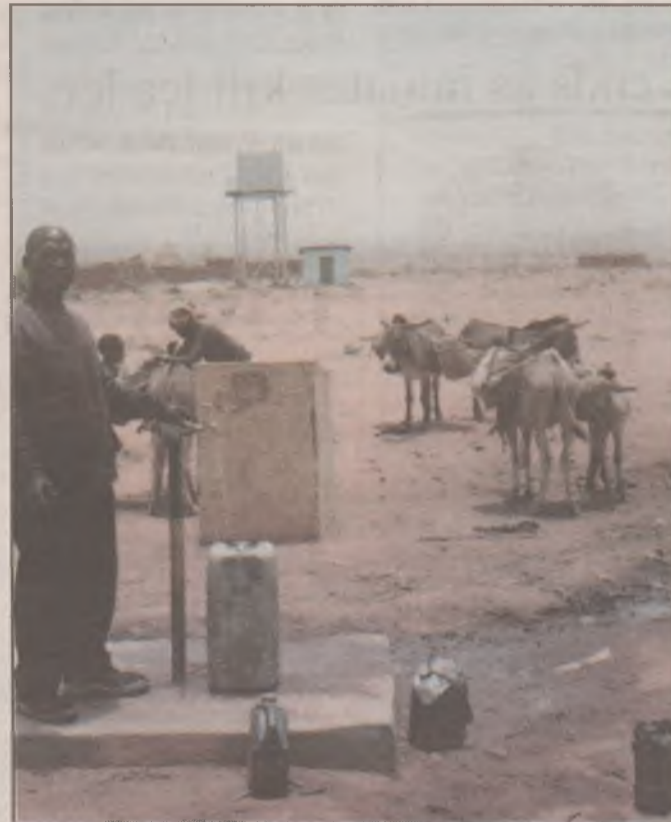
Wuro-Dole Water Scheme initiated and completed by Abubakar Hashidu administration.
