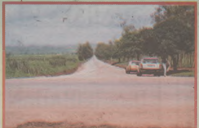
Ta-hoss-Rim Bachit rural road project.
