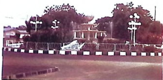
• GRA roundabout, Katsina. New looks
