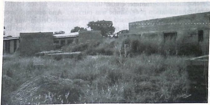
Guma Beach Hotel under construction
