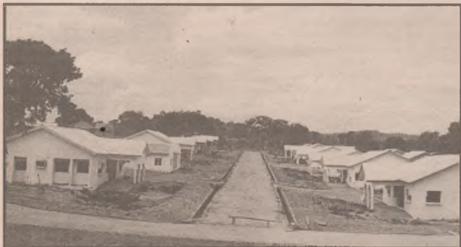
Oba Michael Olobayo 200 housing units along Ganaja Road Lokoja. Another project of Prince Audu's regime
