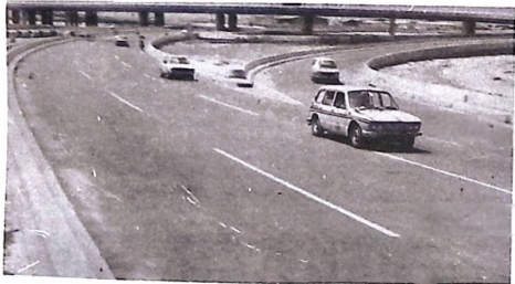
A section of the Lagos Inner Ring Road complex — the largest single contract award so far
