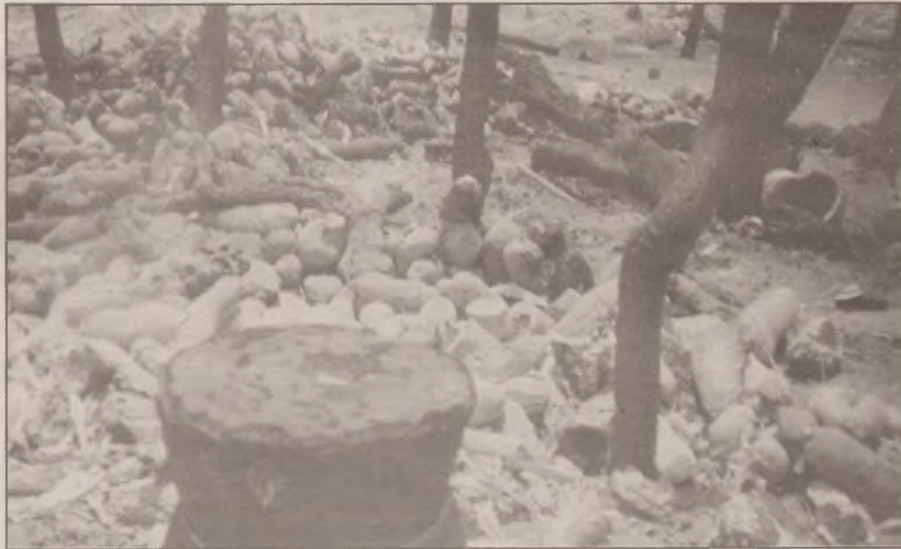
A devastated residence at Kundu
