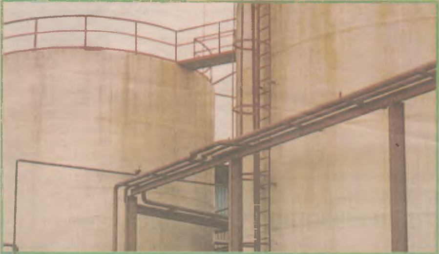
Palm Oil Storage facility at ADAPALM
