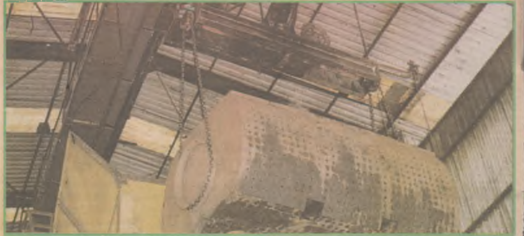
The Palm Fruit cooker at Adapalm Oil Mill, Ohaji being lifted by Crane.
