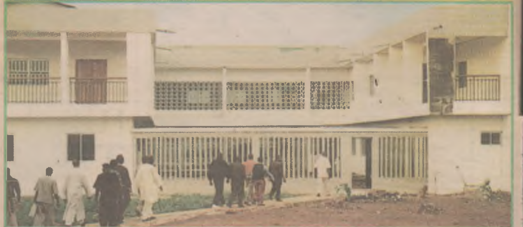
Deputy Governor's Lodge at New Owerri started and completed by Governor Achike Udenwa Administration
