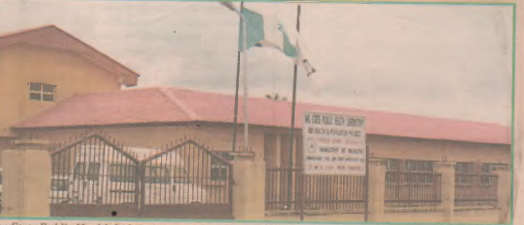
Imo State Public Health Laboratory completed commissioned by Achike Udenwa Administration
