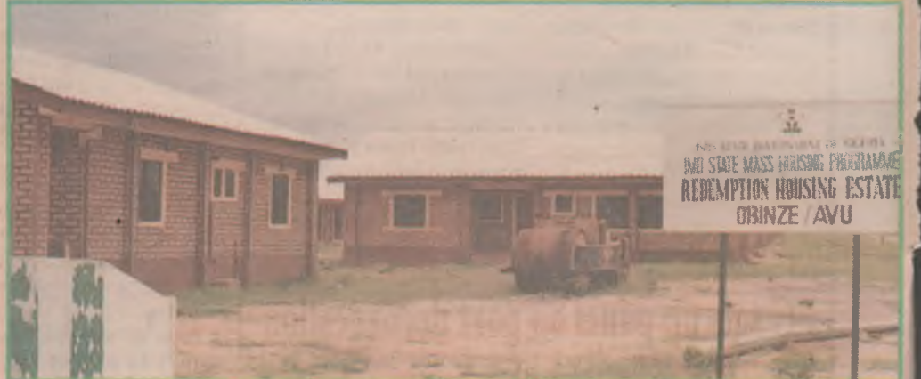
Completed and Commissioned Units of Imo State Mass Housing Programme, Redemption Housing Estate at Obinze/Aru
