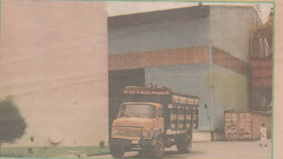
Front view of Adapalm Oil-Mill at Ohaji, Imo State rehabilitated by Chief Achike Udenwa's Administration.
