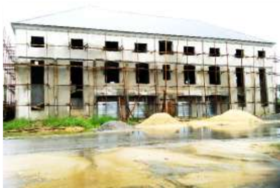
Figure 10: The mixed-use development on 70% completion (finished to roofing)
