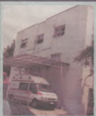
Lagoon Hospital, Lagos
