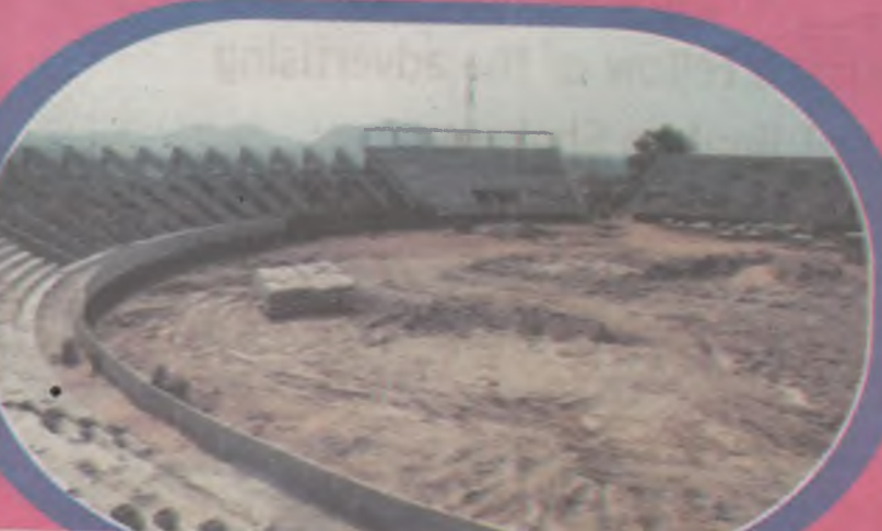
Lokoja International Stadium (under construction)
