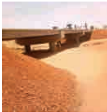
Rehabilitation of NGIBI BRIDGE, Teteba Road, Gulani LGA
