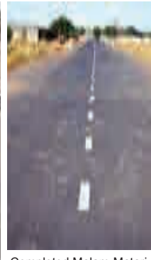
Completed Malam-Matari Road in Damaturu
