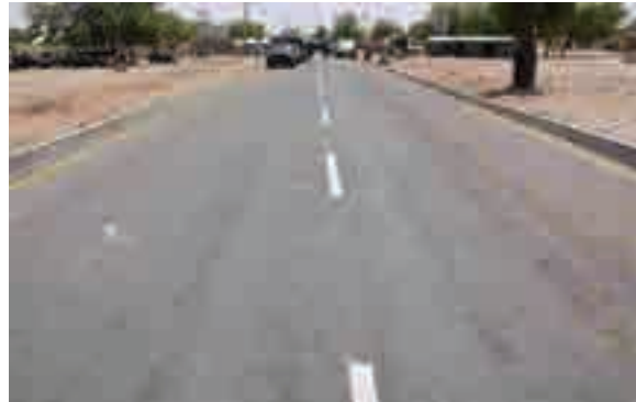
Babbangida Road completed and commissioned
