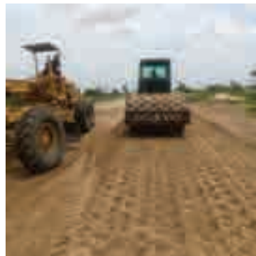
Geidam township road under construction
