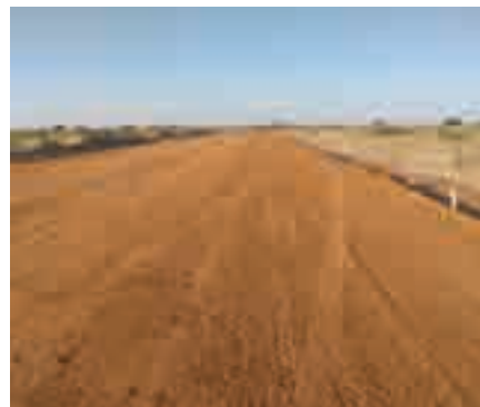
Damagum-Gubana Rd under construction
