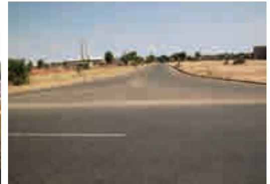
Completed Buni Yadi township road
