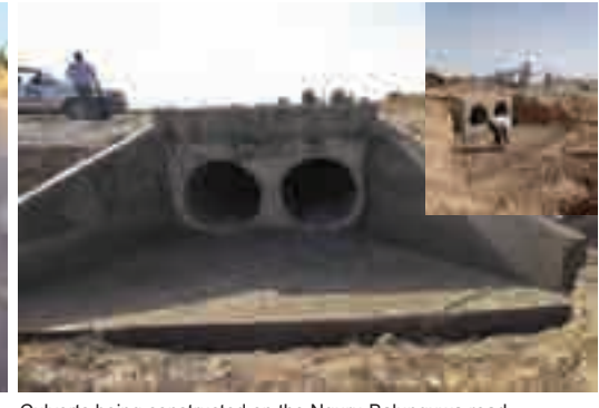
Culverts being constructed on the Nguru-Balanguwa road
