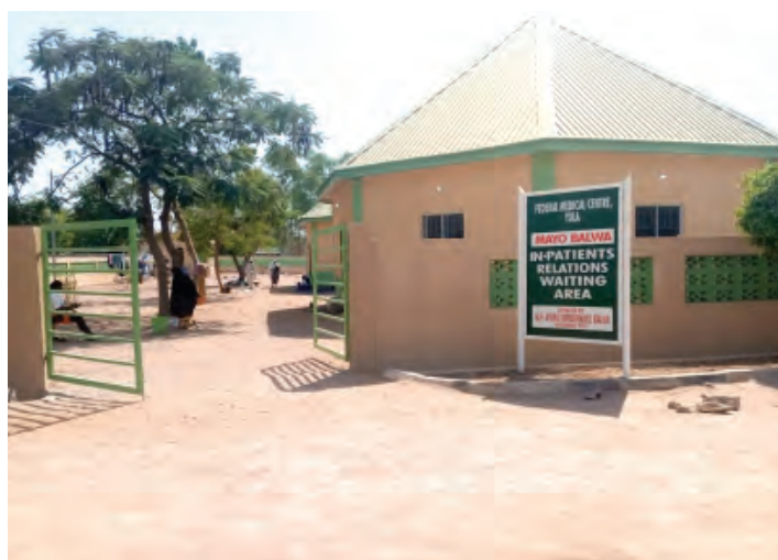
■ The newly completed in-patients' relations building
