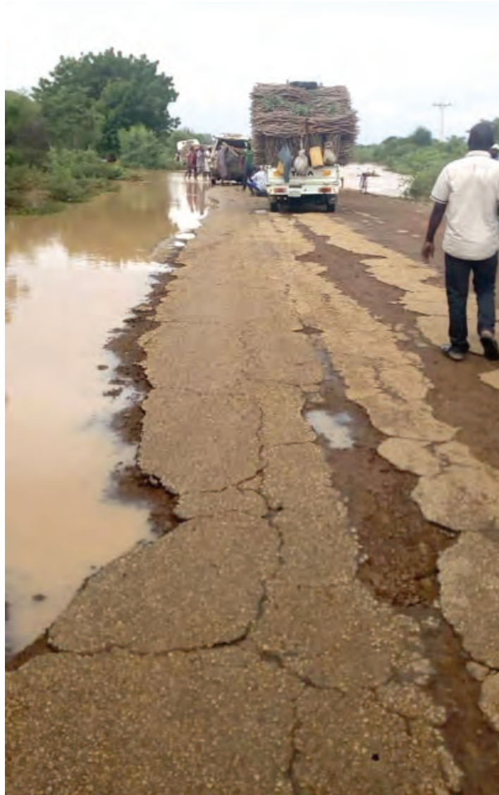
■ A bad section of Tikau-Jajere road in Yobe State
