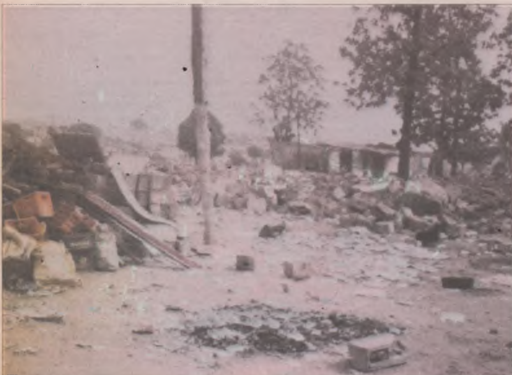
A section of a demolition site at Karmo.
