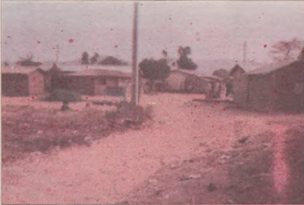
Pegi, a settlement for relocated victims of Idu/Karmo demolition
