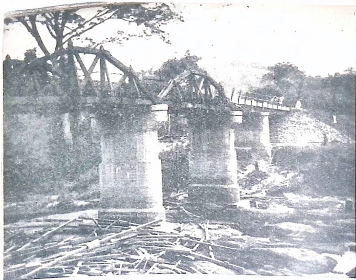
Osse River Bridge.
