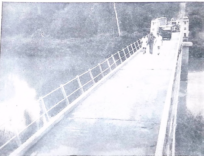
New river bridge in Ijebu Province.
