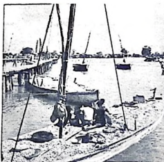
Groundnuts being loaded in the Gambia.
