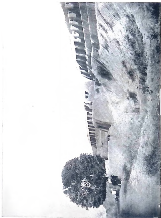
11 The inside of the Kano city wall in 1903. The break in the wall is a re-entrant in which one of the thirteen gates, the Kofar Mata, was set. The outer face of the wall was much steeper, almost sheer, and was protected by a double ditch which was choked, over much of its length, with an impenetrable growth of thorn.
