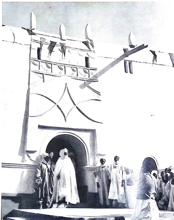
10 The ornamental entrance to the Emir of Yauri's Palace. The building is constructed of sun-baked clay in the traditional Hausa style. In this the roof is supported on arches which are internally reinforced with scantlings cut from fan-palms, the only timber that is not attacked by white ants.
