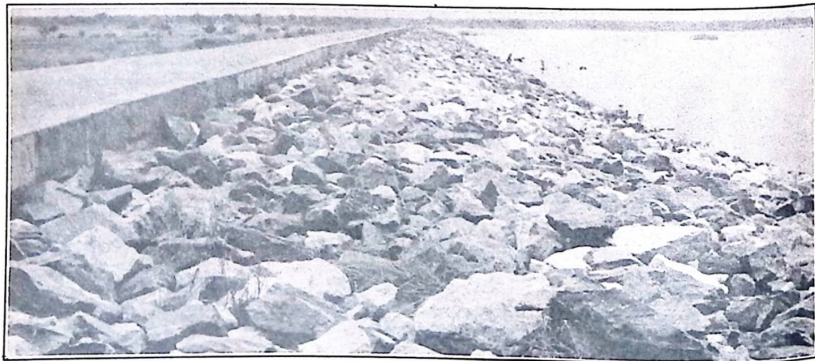
Checking flooding at NRBDA facility.
