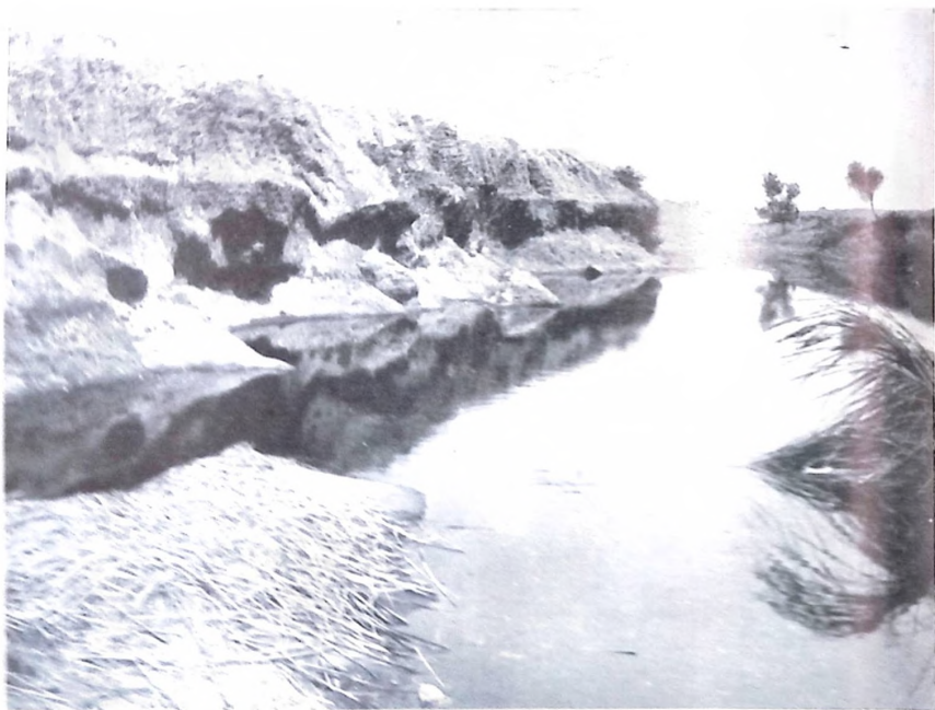
Barrow-pit on outer side of Wall near Kofar Mazugali
