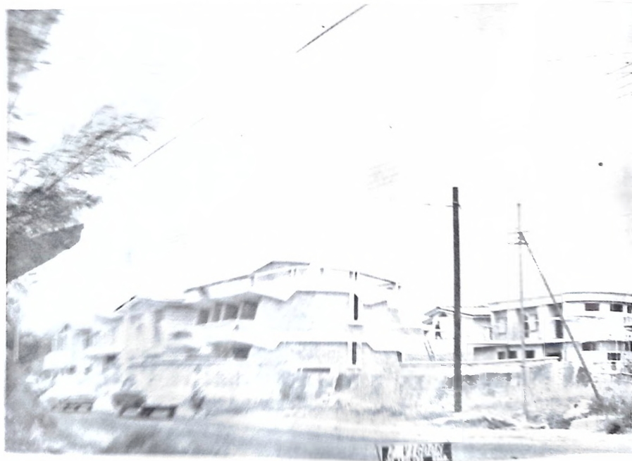
View from a recent house in S.W. Ife
