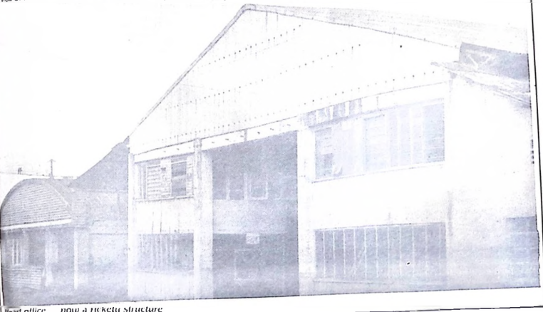
Head office ... now a rickety structure
