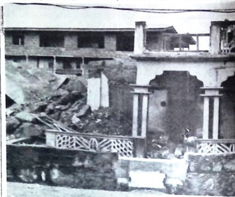
• Devastating effects of recurring Ogunpa floods
