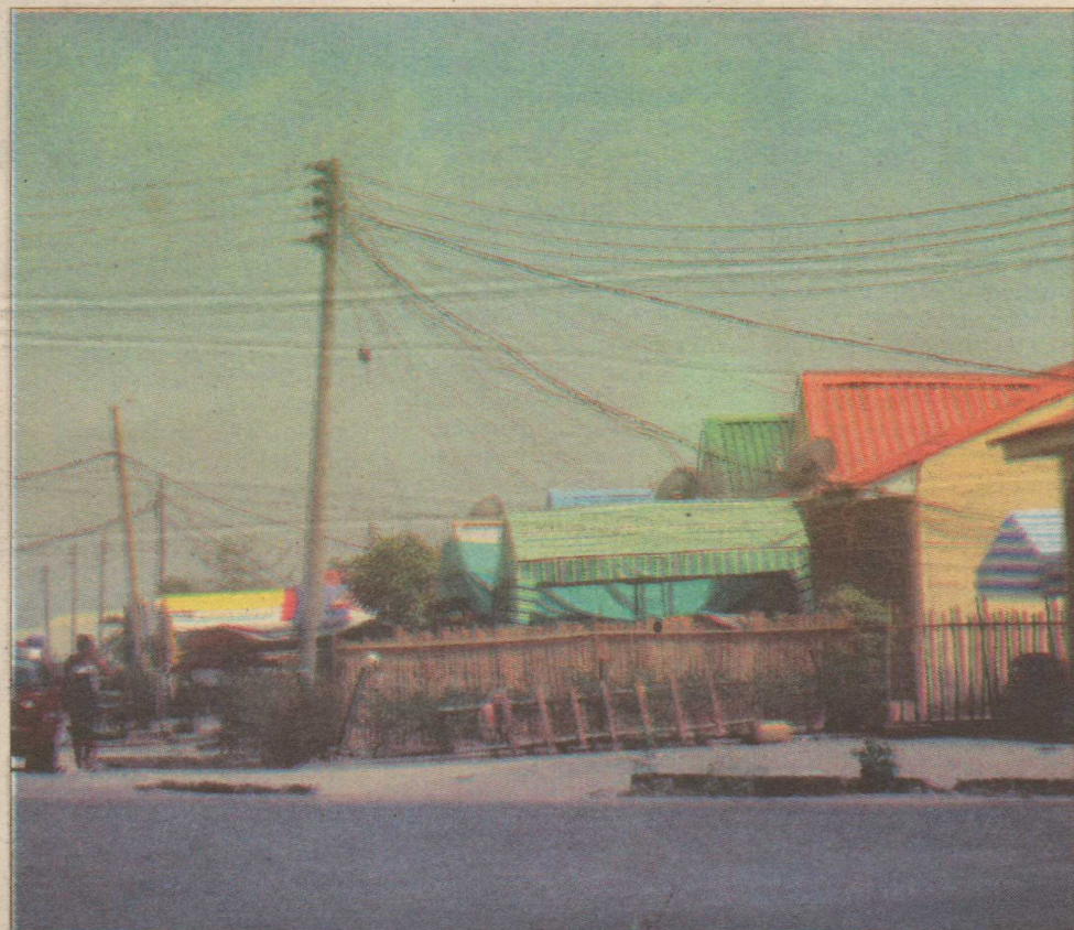
'Illegal' structures at the corner shops
