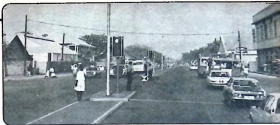
IN THE HEART of the commercial area of Kano: a stretch of the reconstructed H
