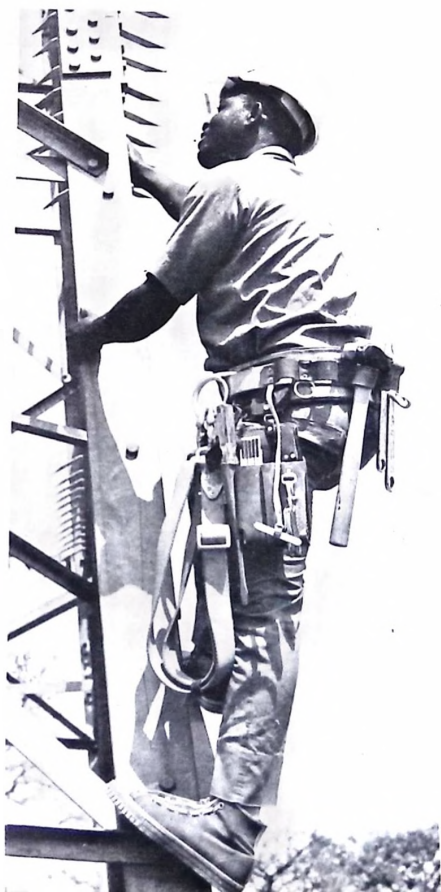
Line maintenance technician on transmission tower
