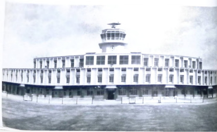
Kano airport terminal
