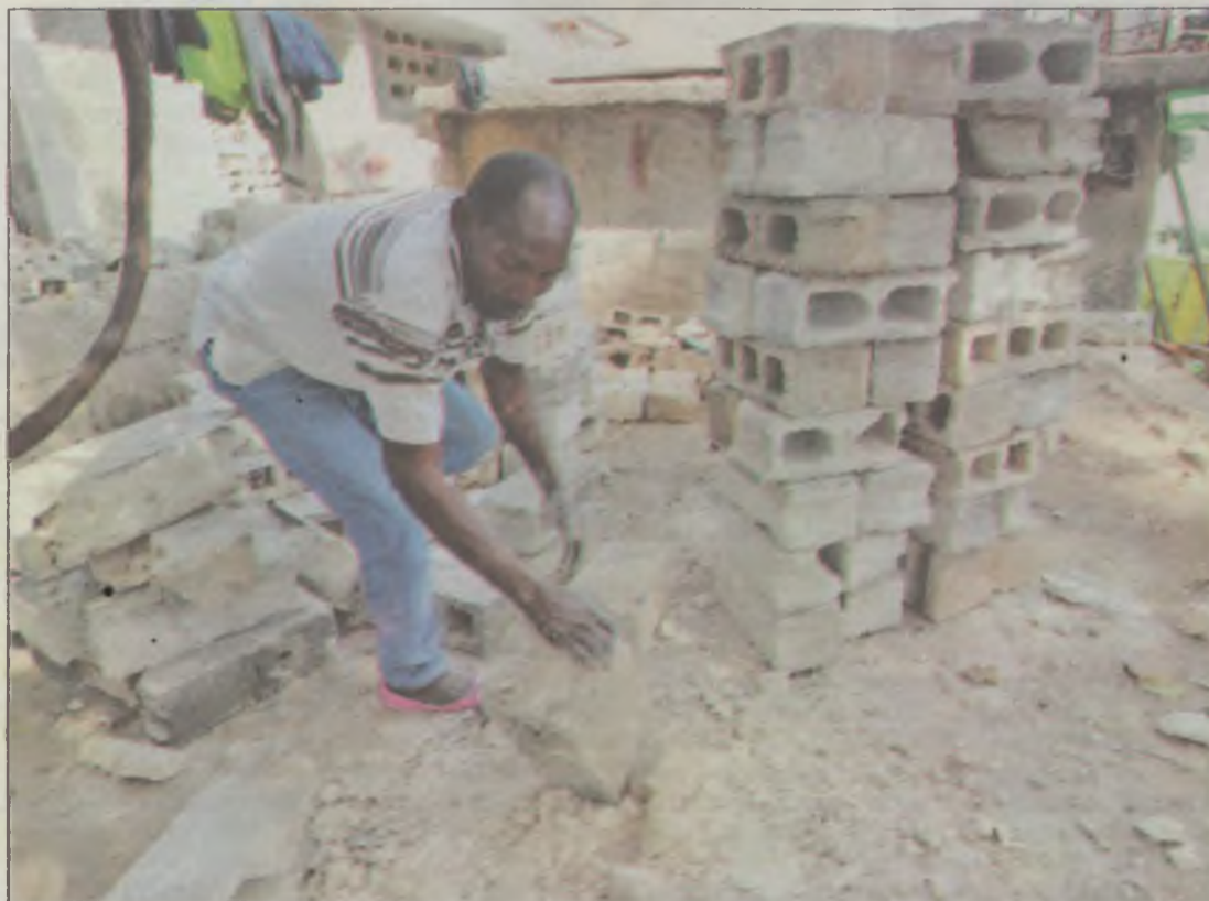
A Haitian man collects usable bricks from a quake-destroyed home to reuse in rebuilding at the weekend
