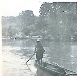
● The other side of Volta Project
