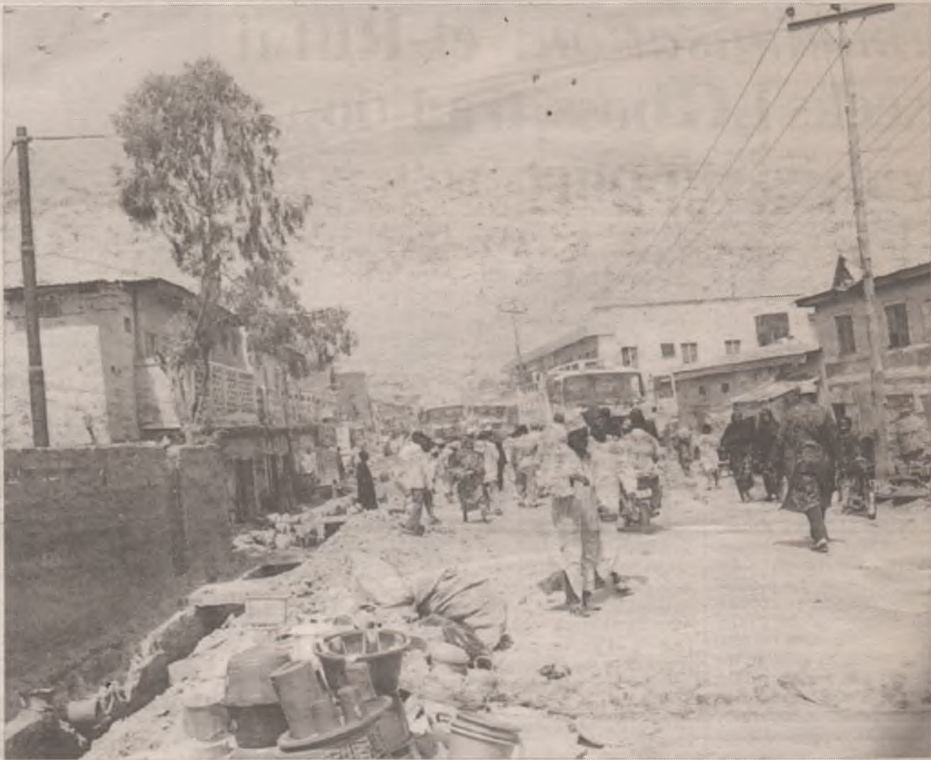
Sterling Nigeria plc returns to Kaduna-Kano expressway to complete their contract. Work has however stopped at the Chiromawa bridge. Pix: Musa Kazaure.
