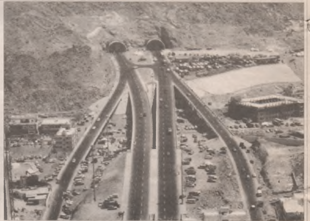
Tunnels are a common sight in Saudi Arabia where the rocky terrain makes it difficult for road and highway construction. This tunnel in Mecca leads to the plain of Arafat, some few kilometres from the Holy city.
