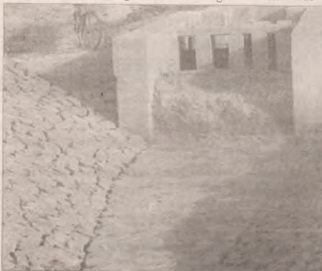
A Downstream trapezoidal canal at the Kano River Irrigation project.
