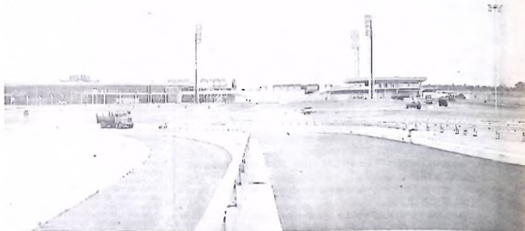
The view of the fair structure from the only way in and out.
