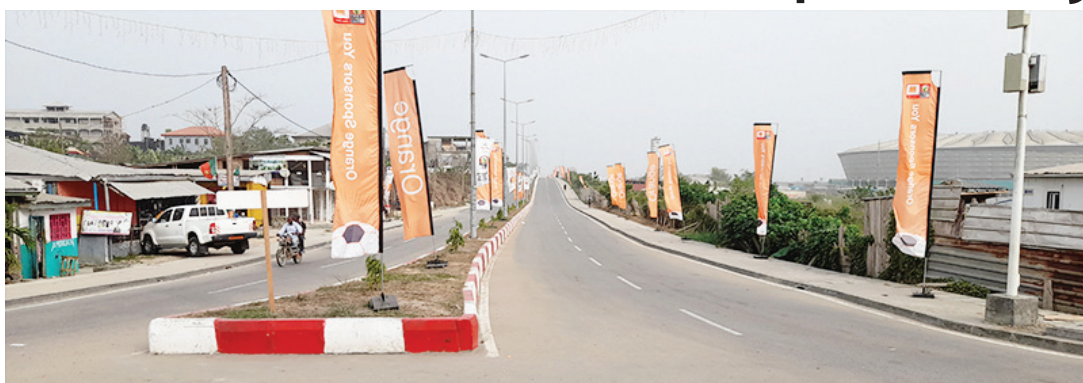
■ Newly constructed road leading to the Japoma Stadium, Doula
