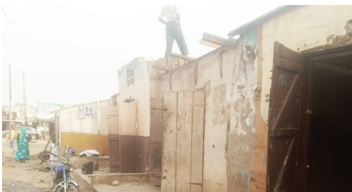
■ One of the sold property with the roof being removed in preparation for demolition at Taiwo Road, Ilorin
