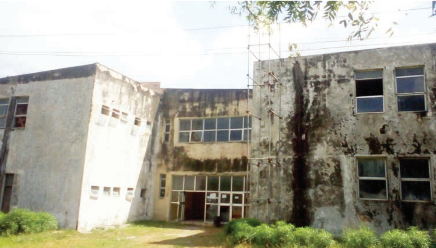
Outside view of the Abubakar Imam Library, Minna, Niger State
