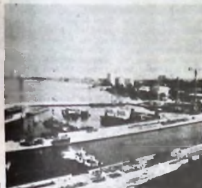
Construction of Naval Dockyard, by Sobat Nigeria Ltd
