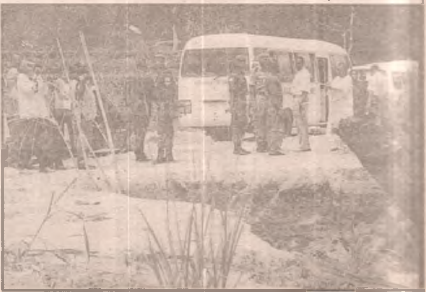
Erosion site at Aba, Abia state
