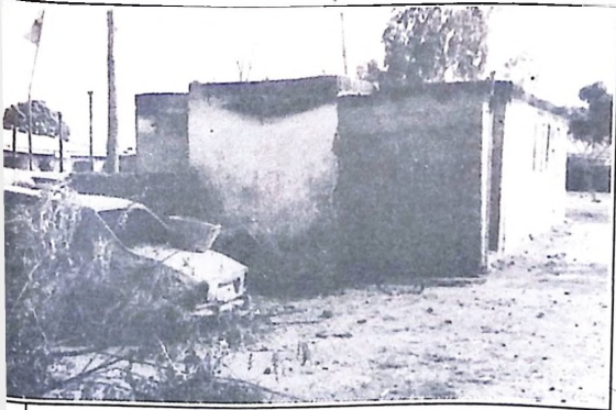
A mosque in Kabala West destroyed
