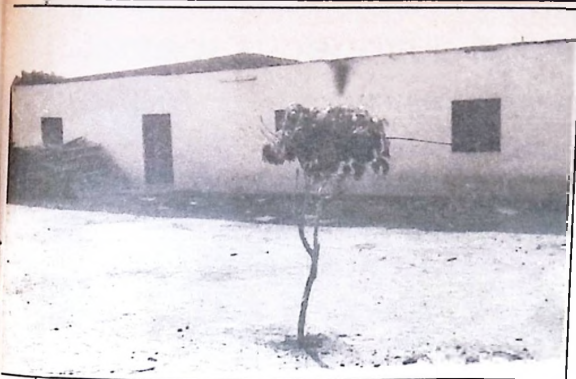
This Islamiyya School at Kabala West also fell
