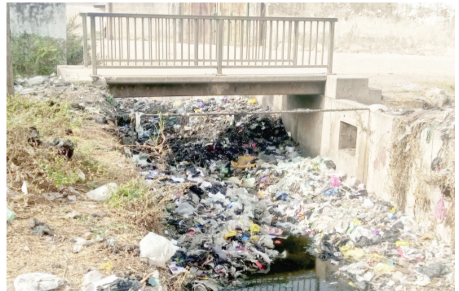
Julius Beggar drainage filled with refuse dumps and human feces in Makera Area of Minna
