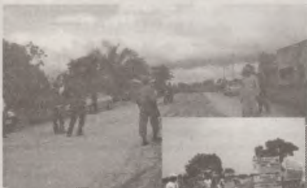
RURAL ACCESS ROADS PROJECTS: MAITZO-KWASU-RANDA RD IN SANGA
