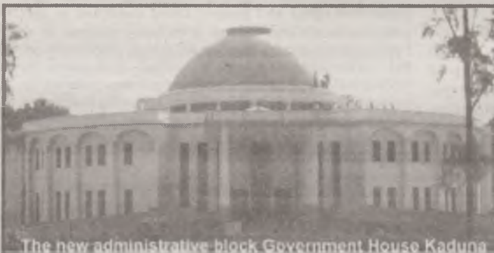
The new administrative block Government House Kaduna
