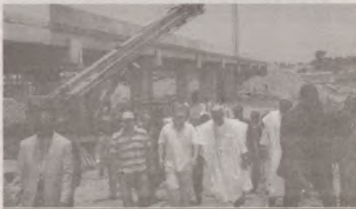
The multi-billion naira Kauru Bridge in Kauru L.G.A.
