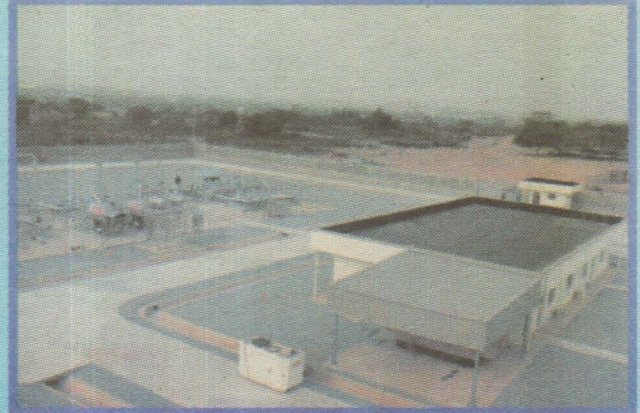
Geregu Gas Station
