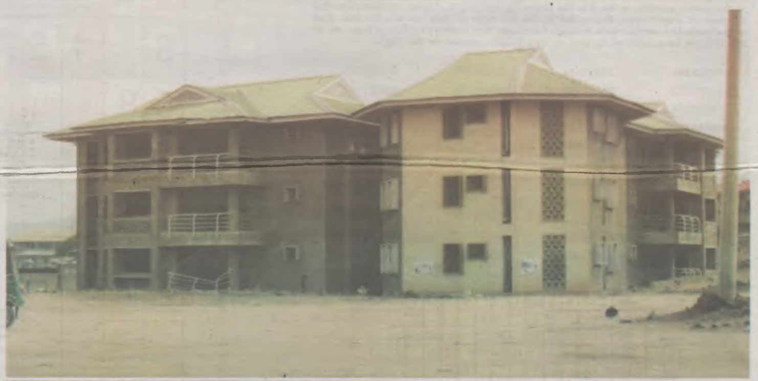
ONE of the block of flats in a yet-to-be-completed estate near Jabi Lake, Abuja
