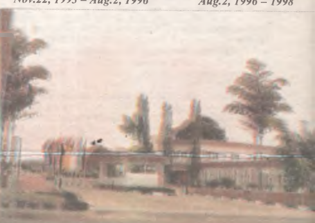
What started in the early 80s as a mere cafeteria services was developed into a full and three stars hotel by the military administration of Col. Fedelis Makka.
