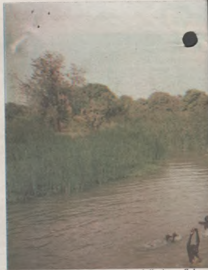
The point of blokage by Typha weeds and siltation at Gubusum
