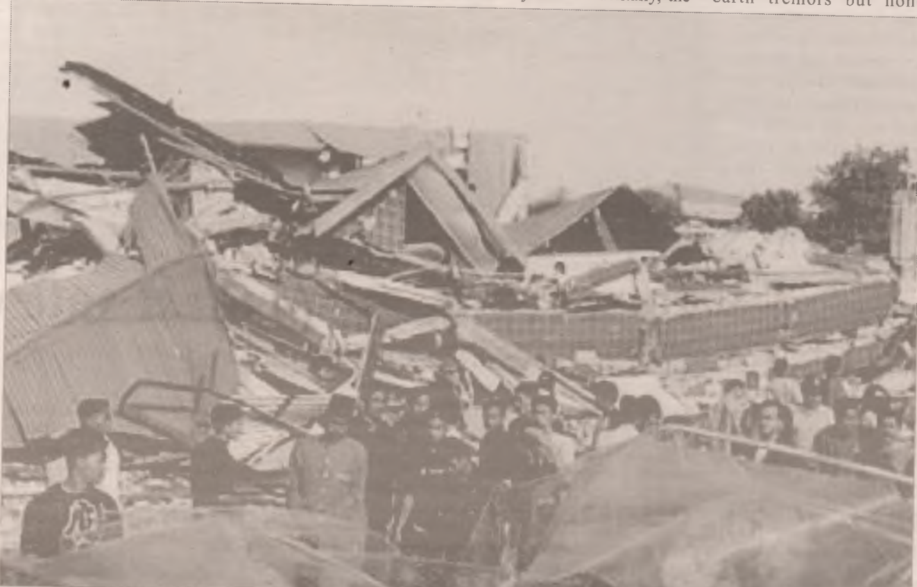
An image showing Acehnese surveying damaged property following the devastating earthquake on December 26, 2004 in Banda Aceh and before the tsunami hit the province. Large parts of Banda Aceh were destroyed by the magnitude 9.0 quake.
