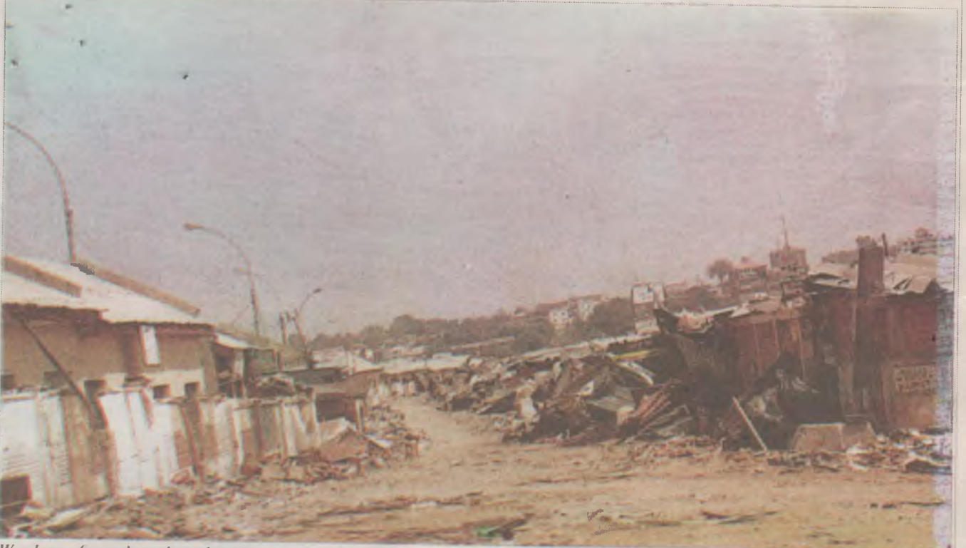
Wreckage of container-shops demolished by the Abuja Environmental Protection Board.
