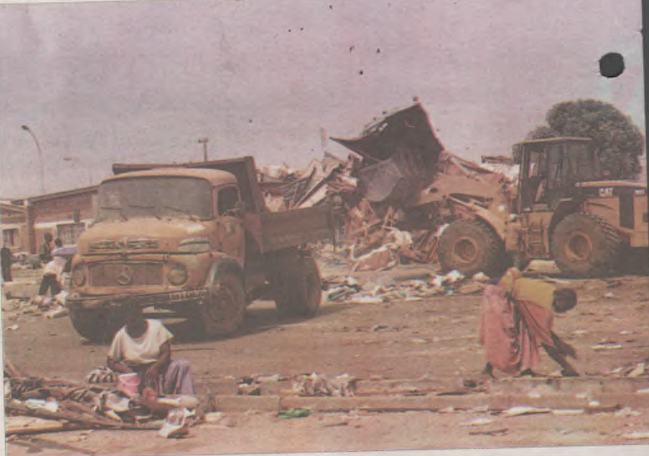
A bulldozer loading demolished container-shops into a truck.
