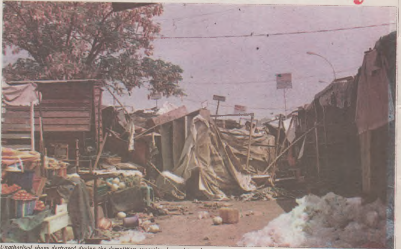
Unauthorised shops destroyed during the demolition exercise, heaped together.
