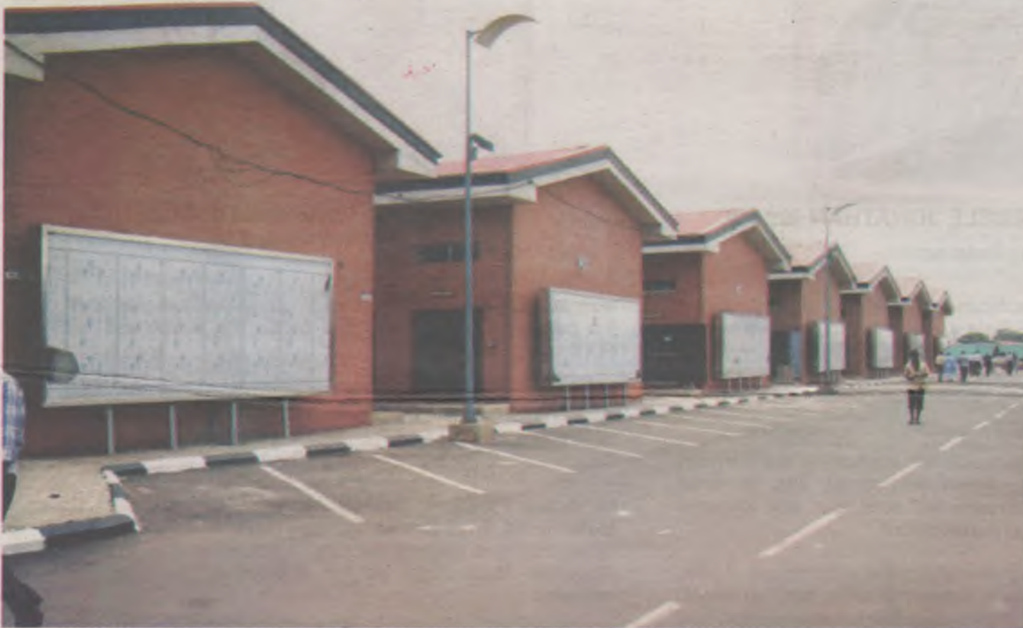
THE Arena shopping complex, Lagos
