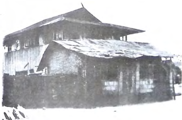
An old 19th Century type of pre-fabricated building (background) A mud and corrugated iron sheet type of building (Fore ground)
