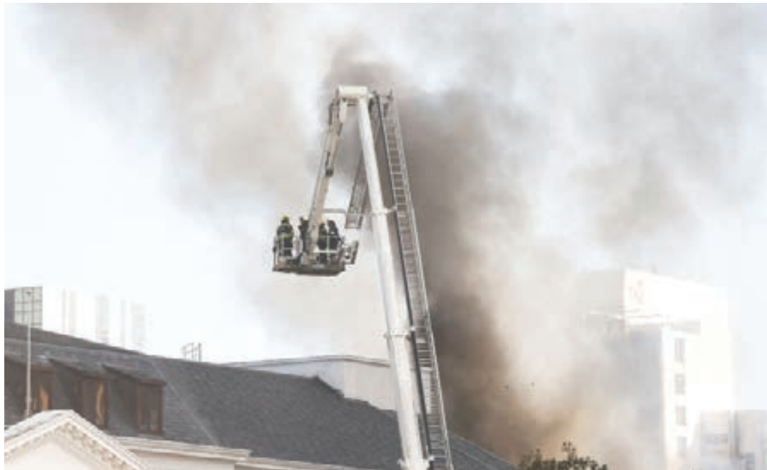
■ Firefighters at the South African Parliament roof in Cape Town during a fire incident yesterday Photo: AFP
