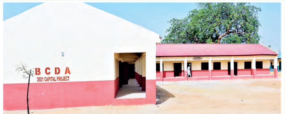
THE BLOCK OF SIX CLASSROOMS CONSTRUCTED BY BCDA AT UMARU ILLALU MODEL PRIMARY SCHOOL, BADARIYA, BIRNIN KEBBI, KEBBI STATE.
